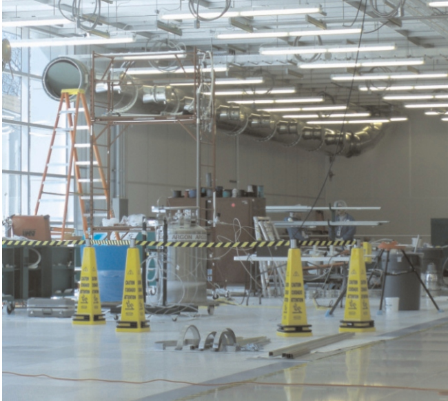
PSP® duct installation at NonoFab 300 South Annex, Albany Nanotech, NY
