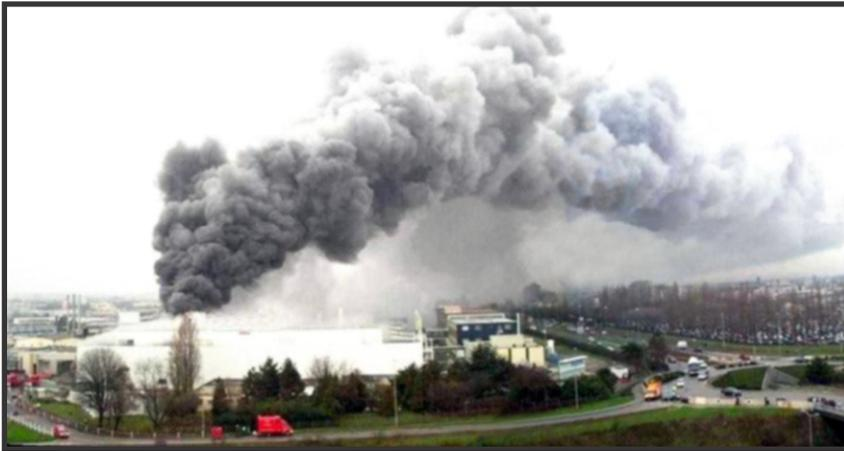
Building loss in excess of \$400 million USD, exclusive of production and downstream interdependency losses. A contributing factor to the spread of the fire was the use of plastic exhaust duct.
