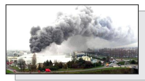
Building loss in excess of \$400 million USD, exclusive of production and downstream interdependency losses. A contributing factor to the spread of the fire was the use of plastic exhaust duct.
